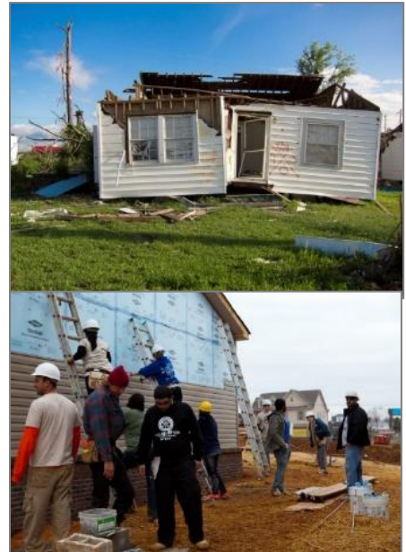
Above: A disaster-destroyed home. Below: Volunteers repair a home.
