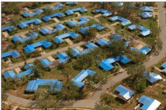
US Army Corps of Engineers' Blue Roof Program helps to prevent further damage to structures as a result of Hurricane Katrina in Biloxi, Mississippi.
